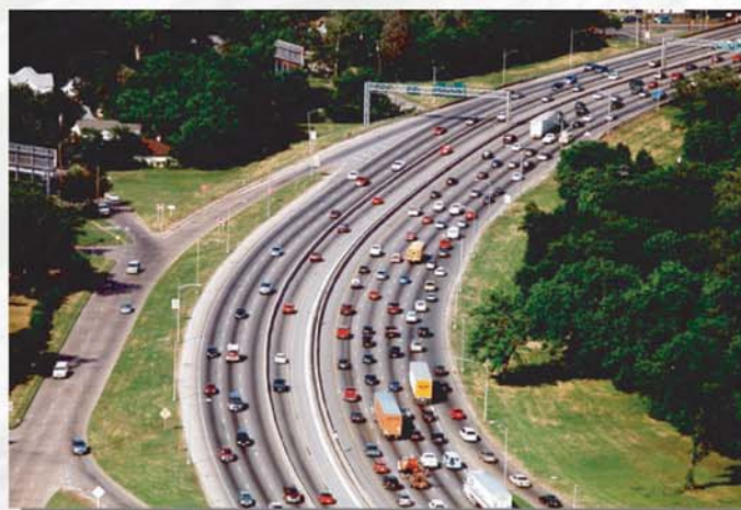
Traffic Congestion on Interstate Highway 30
